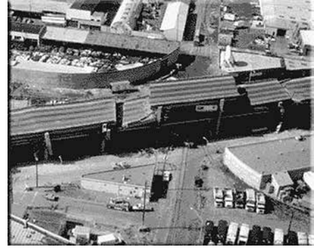
Aftermath: collapsed freeway
