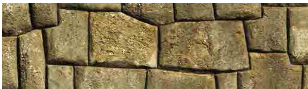
Tightly wedged stones
