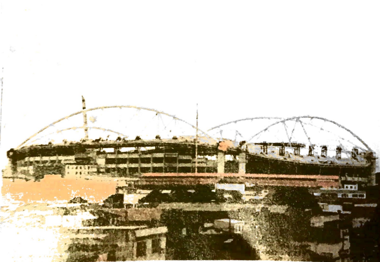
3.78 Estádio Nilton Santos required extensive renovation where it could be used for the 2016 Olympic Games as a wall in the stadium had collapsed in 2008, and after a forced closure in 2013 when it was found the structural integrity of the roof was sub-standard.
