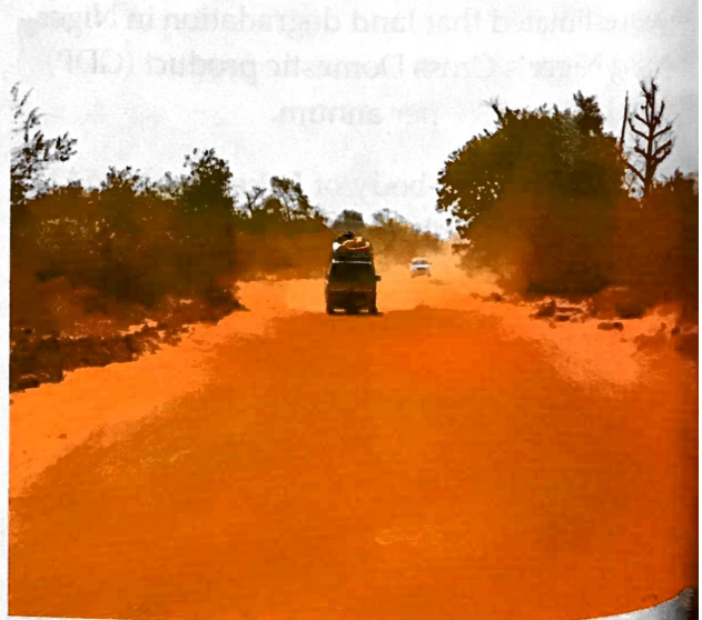
2.88 Wind-blown sand covers the international highway between Dosso to Gaya that connects Niger with Benin.
