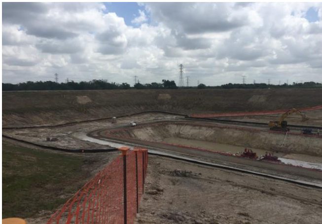
Photograph 1: The new flood dam gate being built
