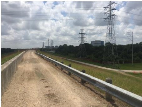
Photograph 5: The access road located on top of the reservoir wall.
