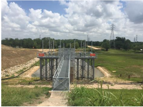
Photograph 3: The Flood Gates
