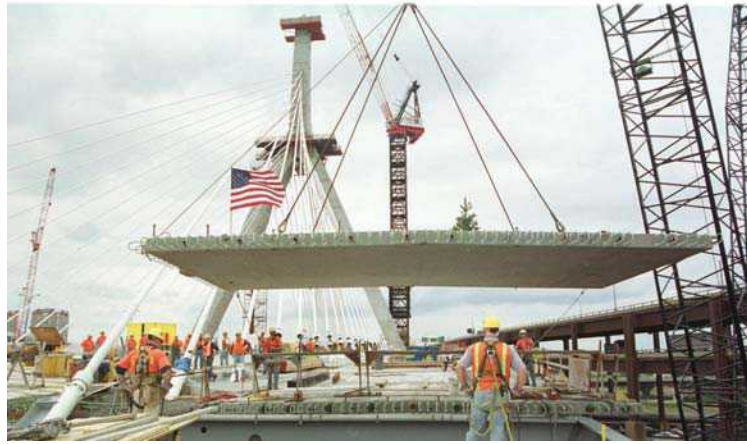
Construction of the Zakim Bunker Hill Bridge, Boston, Massachusetts
