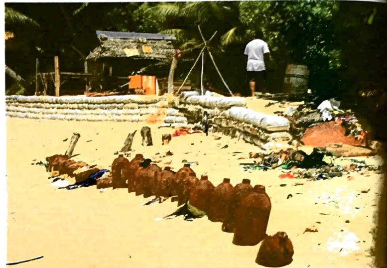
6.27 A sandbag-and-cement seawall (background) has been partially washed away, so local residents have responded by erecting a barrier of old, disused metal gas bottles to absorb wave energy. This seawall is in Teaoaraereke village.
