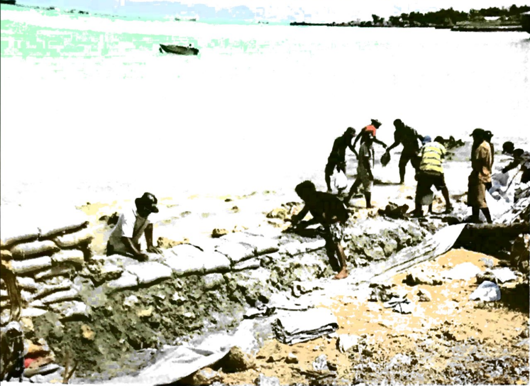
6.33 A new seawall being built on Betio Island.
