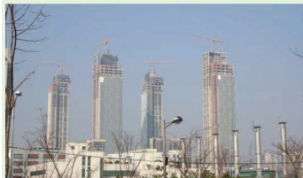
Figure 18 High-rise buildings in Seoul
