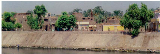
Figure 8 Low-income housing on the banks of the river Nile, Egypt
