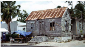
Figure 3 Poor-quality housing in Oisins, Barbados
