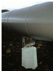
Figure 14 Pipeline on rollers
