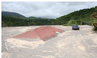
Figure 11 A building buried by a mudflow in Plymouth, Montserrat – one of the disadvantages of tectonic activity
