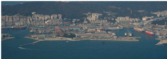
Figure 21 Aerial view of Hyundai shipyard in Pusan, Korea
