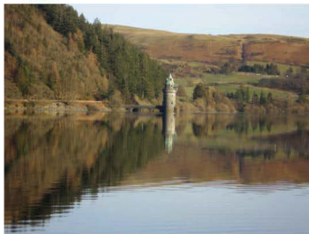
Reservoir with water tower in Wales
