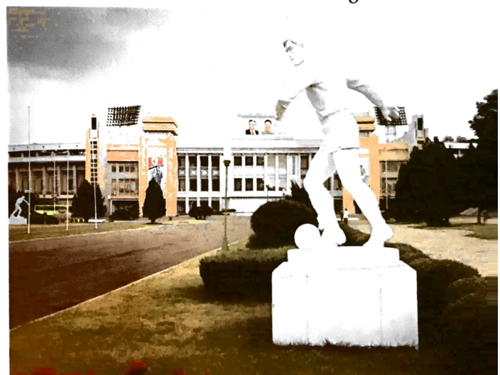
3.56 Kim Il Sung Stadium in Pyongyang, North Korea, was built in 1969, and is used regularly to host qualifying rounds of the FIFA World Cup. It is also used extensively throughout the year for soccer matches, and it is the site of the start and finish of the annual Pyongyang Marathon.
